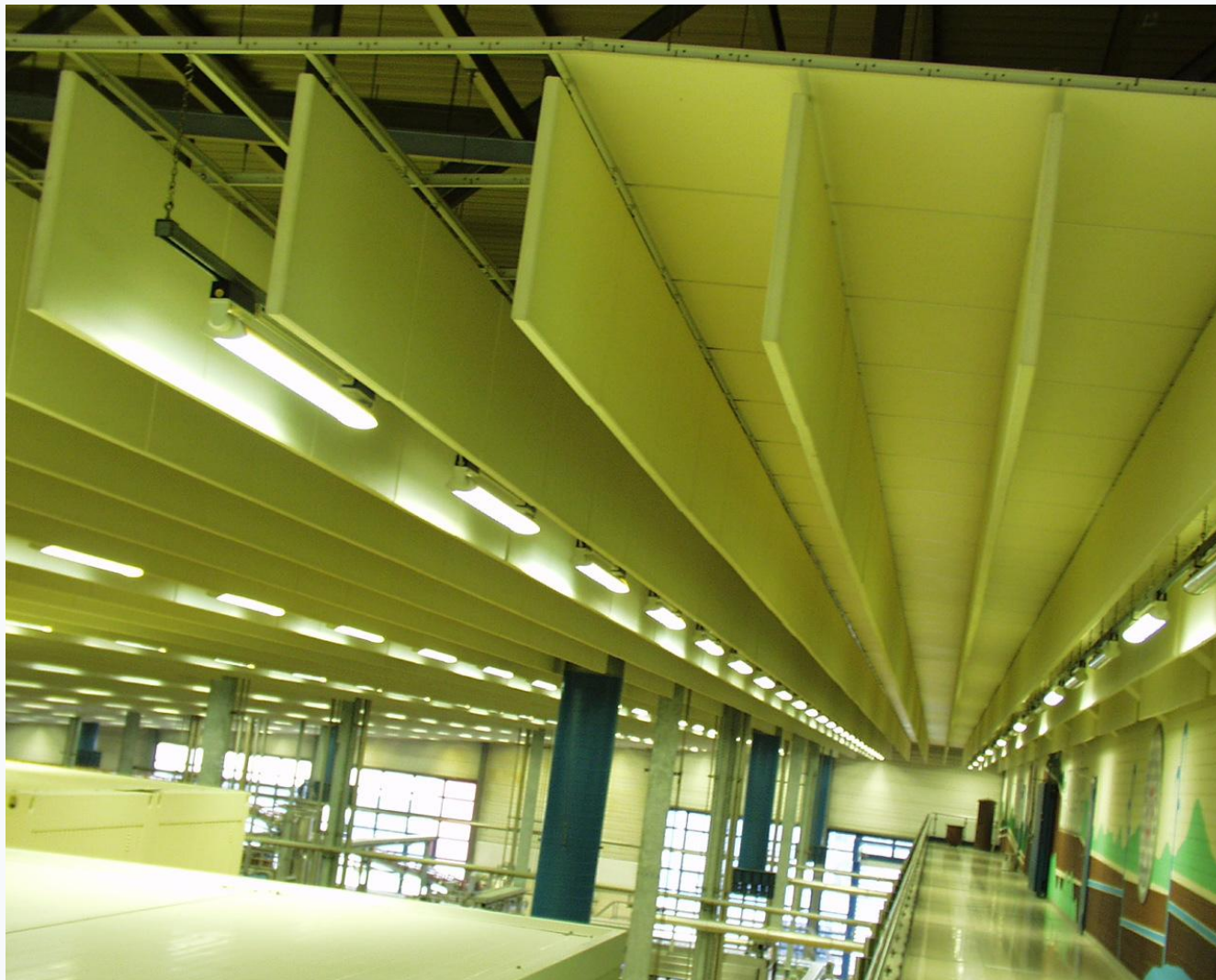
Absorbing baffle system at the ceiling
