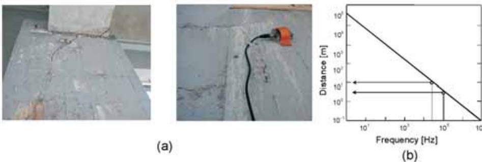
Fig. 3 : Cracks in the P<sub>1</sub> pier and the applied sensor (a). Relationship between signal detection distance and signal frequency (b).
