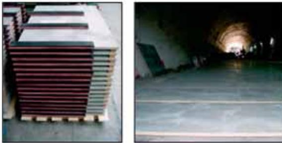
Fig. 16 : Fibre-cement boards with CDM-DFSA resilient strips and installation
