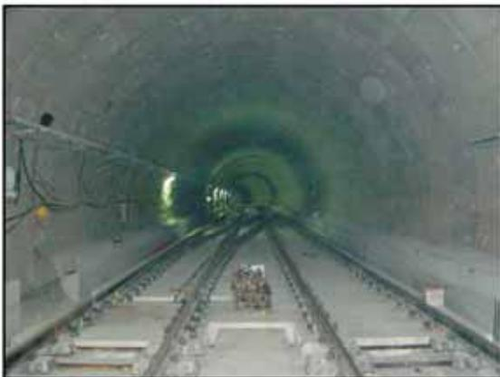
Fig. 17 : Finished installation of FST
