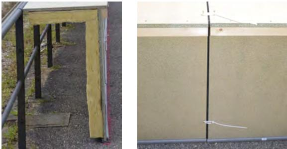
Fig. 3 : Views of the low height barrier prototype. Left : cross section. Right : joint system between elements
